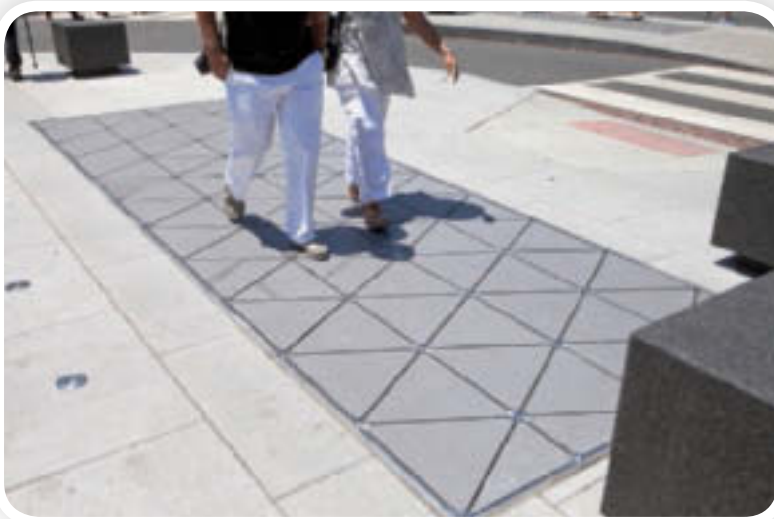
Each step on this experimental sidewalk captures energy of motion and converts it into electricity.
